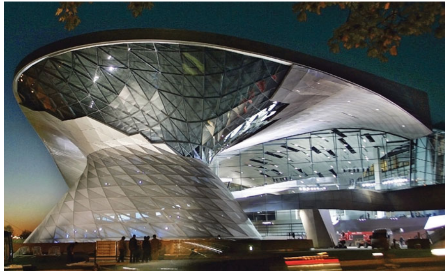
The Austrian firm Coop Himmelb(l)au designed this building, called the BMW Welt, to house showrooms and a museum for BMW automobiles in Munich.
